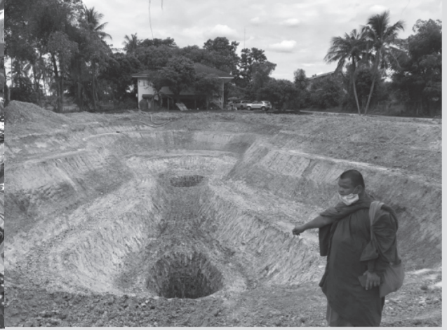
Two holes dug deep enough to reach the aquifers. This will allow water to stay cool all year.
